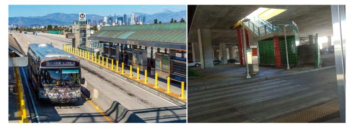
Access from above: San Diego MTS Rapid 235 line at City Heights Station, showing the freeway median station underneath the local roadway used for passenger access.
